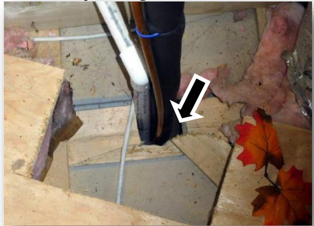
Seal air infiltration at gable end
