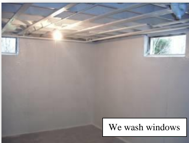
Basement with sealed walls and ceiling
