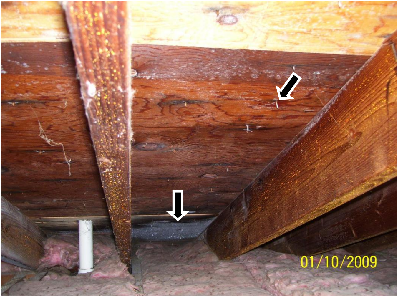
Frost forming on the sheathing and roofing nails.
