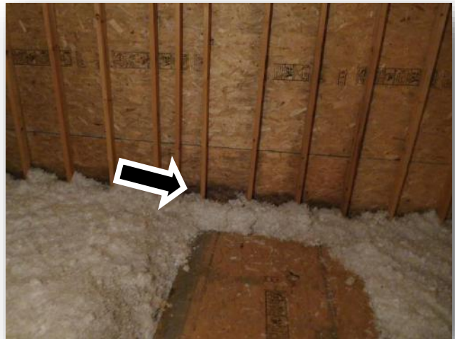
Seal air infiltration at gable end
