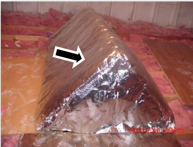
Note wet roof sheathing from improper air sealing and an underperforming ridge vent.
