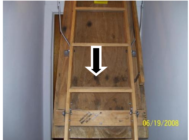
Condensation drip marks on the insulation and the attic staircase.
