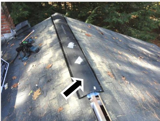
Install a collapse resistant ridge vent
