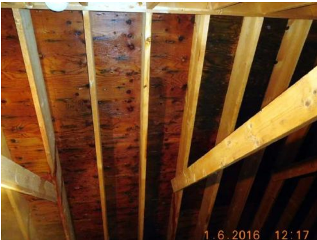
Note wet roof sheathing from improper air sealing and an underperforming ridge vent.
